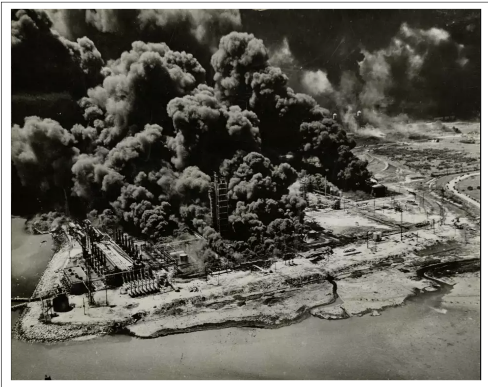
Figure 3-3. A styrene plant became a roaring inferno on April 16, 1947, in Texas City. Hundreds of other fires started in areas where petroleum was stored. Source: the Houston Chronicle. 6
